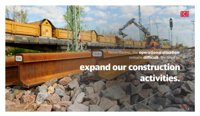
An extensive program to inspect and upgrade ties will account for part of the higher construction volume. This preventive program will involve the replacement of some 480,000 concrete ties this year – in a normal year, we replace around 80,000 ties.
