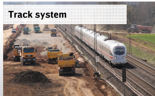
Increased construction activity
