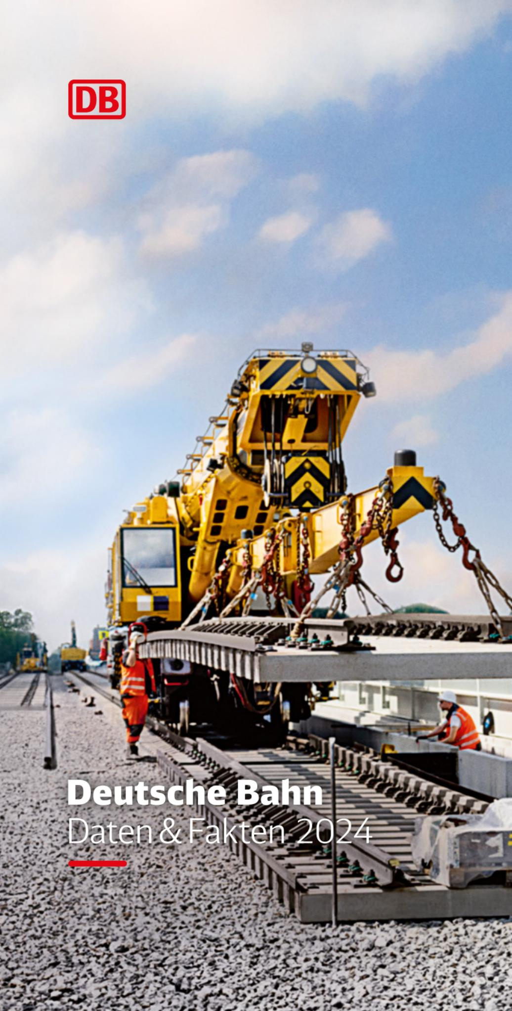
A large yellow and black crane is lifting a long, heavy concrete rail track section onto a gravel bed. Two workers in orange safety vests and white hard hats are visible, one standing near the crane and another working on the track. The scene is set outdoors under a blue sky with scattered clouds.
